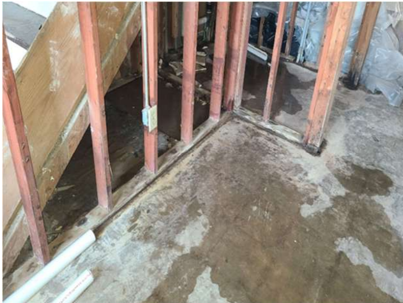
Photo 4: Lower living room framing is rotten. Standing water present.
