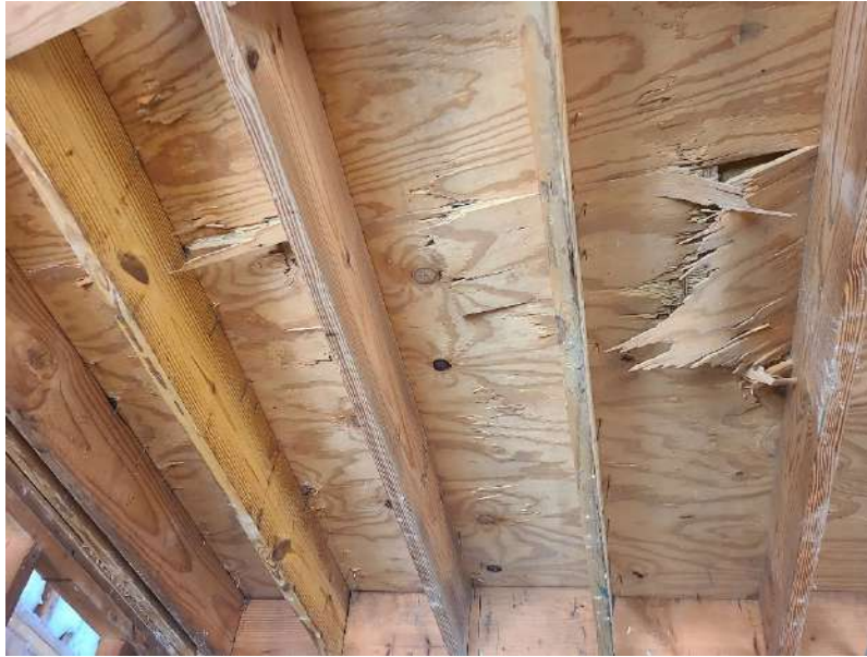
Photo 1: Plywood on second floor is broken.
