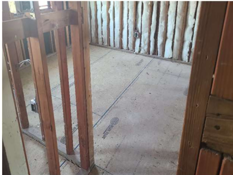
Photo 6: New subflooring has been installed on the second floor.
