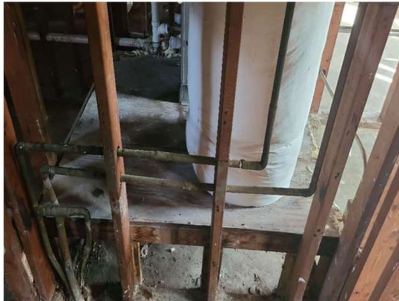
Photo 2: Framing and plywood under hot water heater is rotten.
