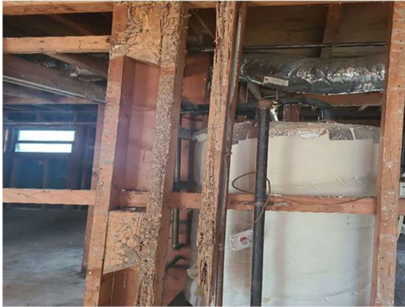
Photo 1: Evidence of termite damage in wall studs near the hot water heater.
