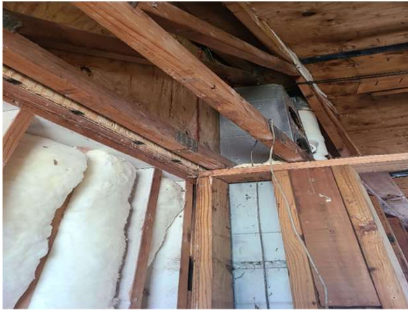
Photo 5: Bottom chord of truss is cut.
