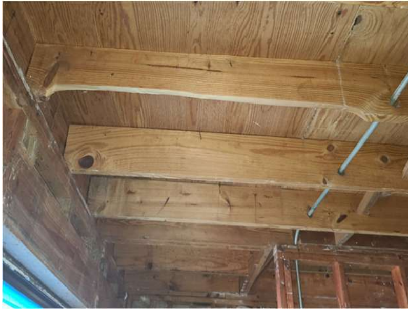
Photo 3: Section of floor joist missing.
