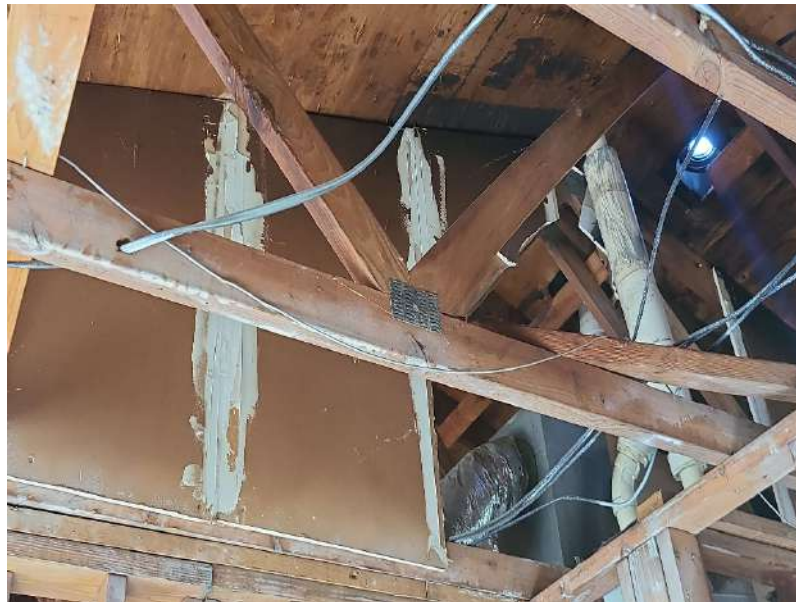
Photo 4: Truss chord splitting at splice plate.
