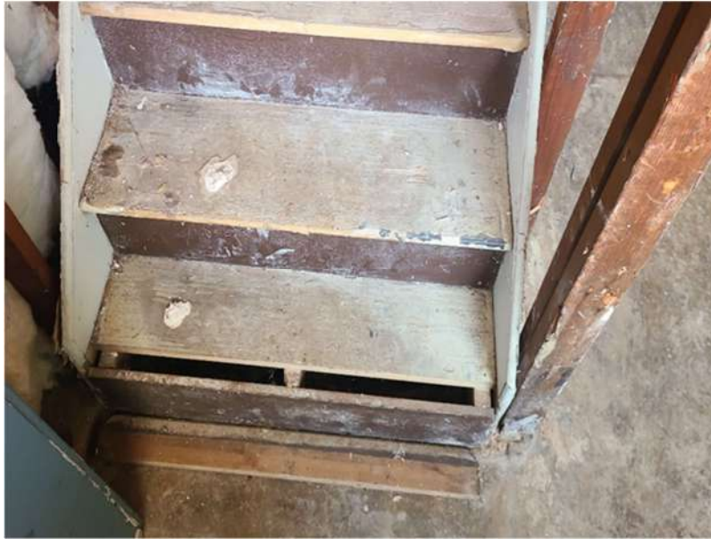
Photo 5: Broken stair tread.
