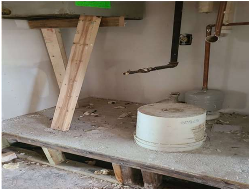
Photo 2: Plywood under hot water heater was replaced.
