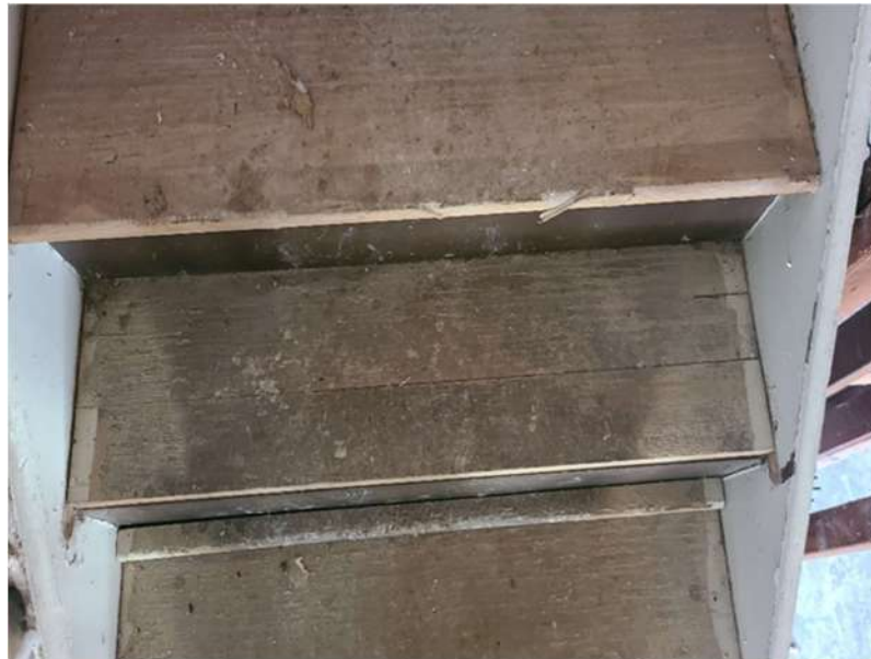
Photo 6: Broken Stair tread.
