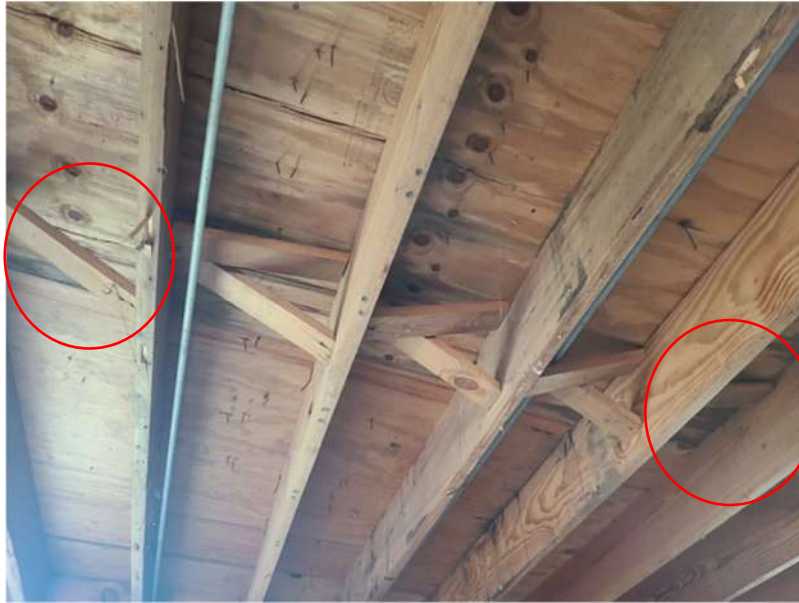
Photo 3: Cross bracing between joists missing in two spots.
