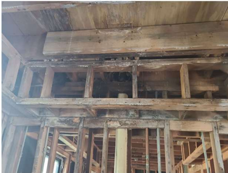
Photo 2: Upper framing in kitchen area is rotten.
