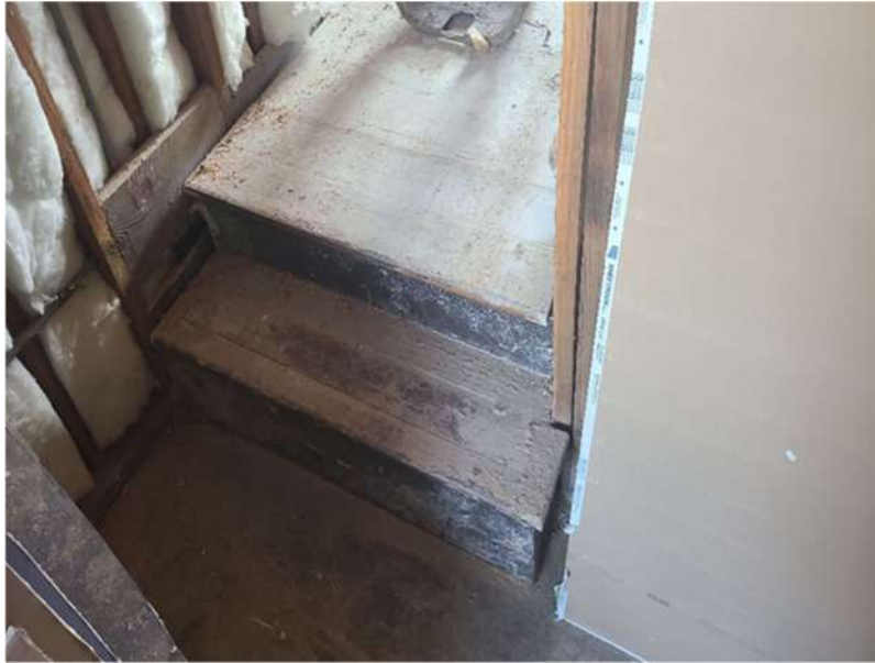
Photo 5: Broken stair tread.
