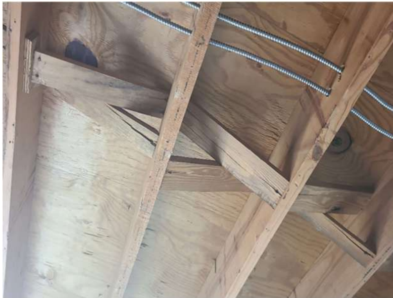
Photo 2: Floor joist cross bracing is cracked.
