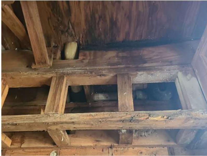
Photo 3: Upper framing and plywood above kitchen area is rotten.
