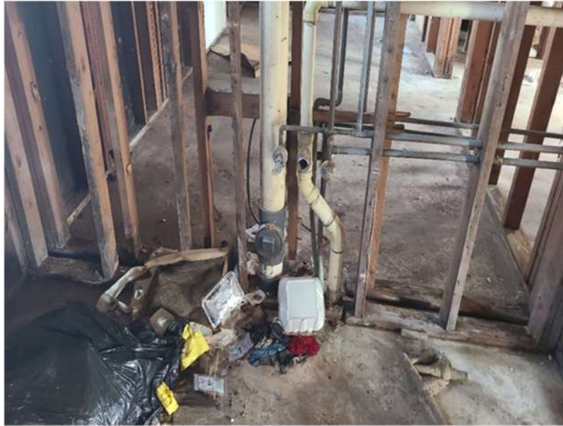
Photo 1: Lower framing in kitchen area is rotten.
