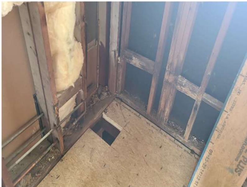
Photo 6: Lower framing in second floor bathroom is rotten.
