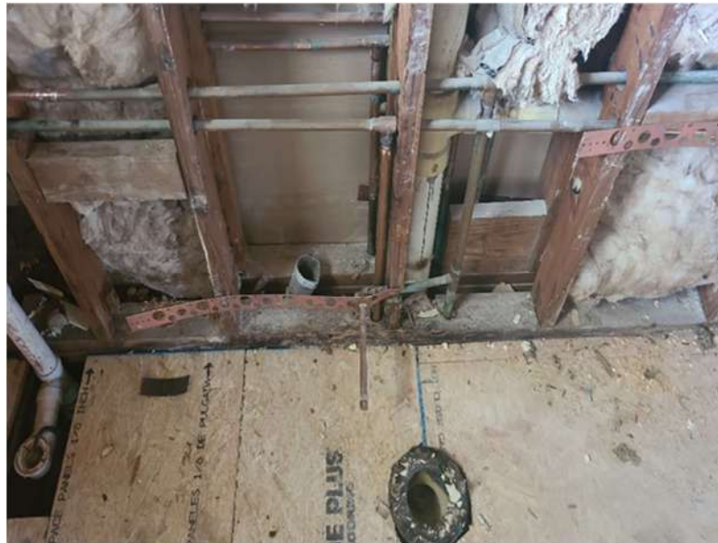
Photo 8: Lower framing in second floor bathroom is rotten.
