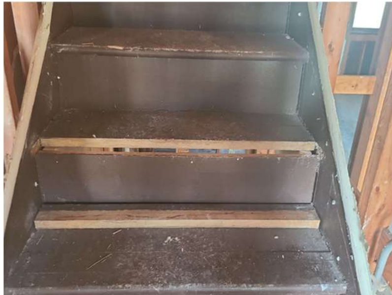
Photo 6: Broken stair tread.
