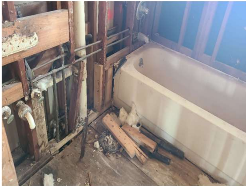
Photo 7: Framing around the bathtub has been partially replaced. Judging from the rotten framing in the kitchen below, further framing will likely need to be replaced behind the bathtub.
