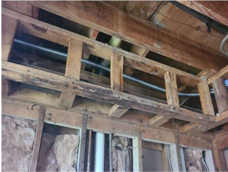
Photo 3: Upper framing in kitchen is rotten.
