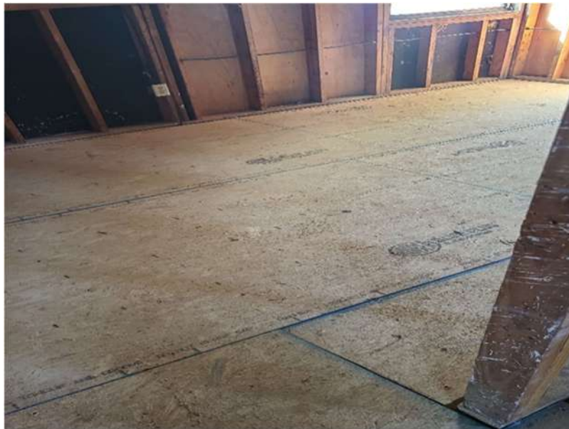
Photo 4: New sub-flooring installed on the second floor.
