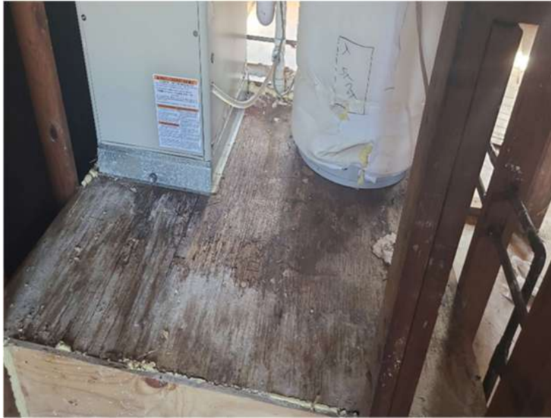
Photo 3: Plywood under hot water heater is rotten.
