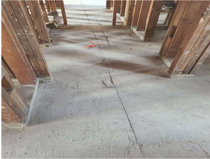
Photo 7: Plywood on second floor was broken in multiple areas.
