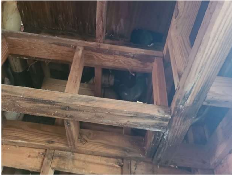
Photo 5: Upper framing in kitchen area is rotten.
