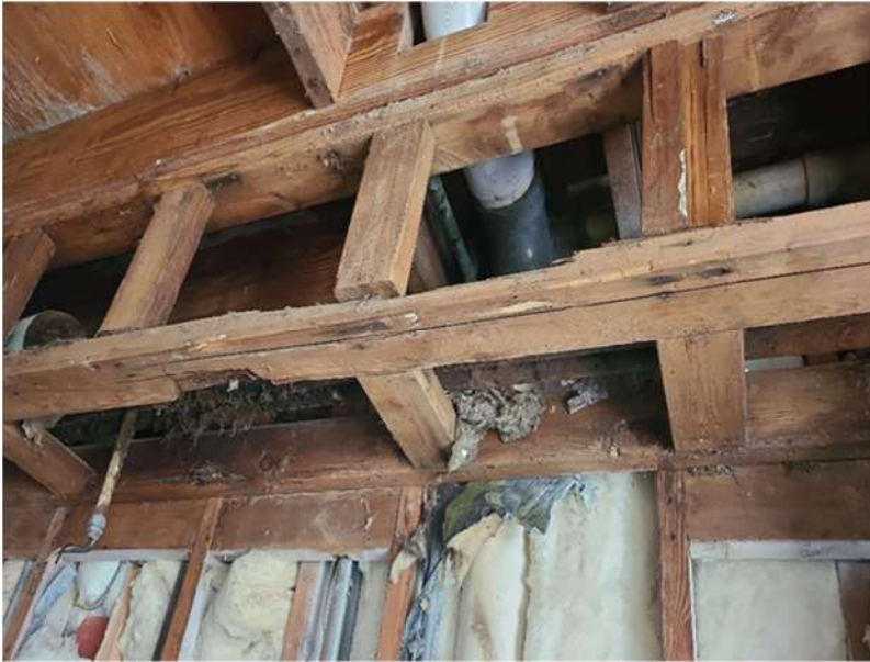
Photo 1: Upper framing in the kitchen is rotten.
