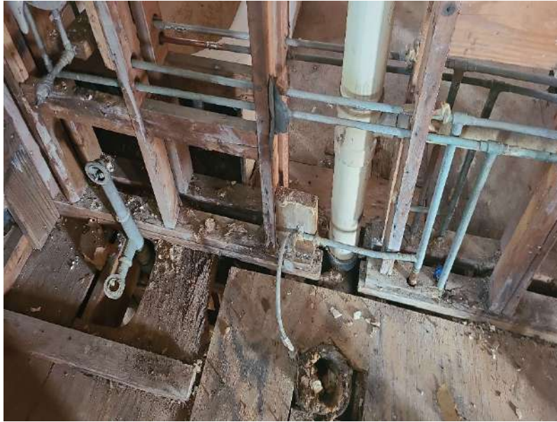
Photo 3: Lower framing and plywood in the 2 nd floor bathroom area is rotten.
