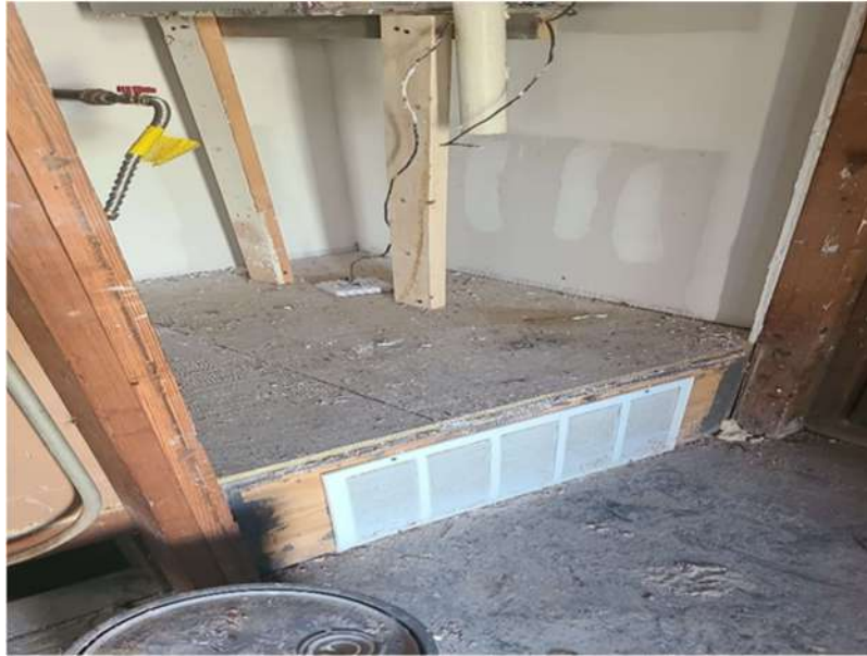
Photo 1: Hot water heater framing has been replaced. Drywall has been installed.
