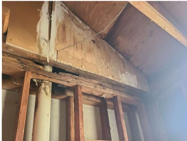
Photo 8: Upper framing in bathroom area is rotten.
