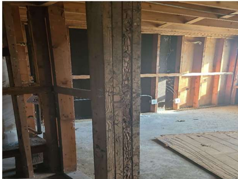
Photo 2: Termite damage.
