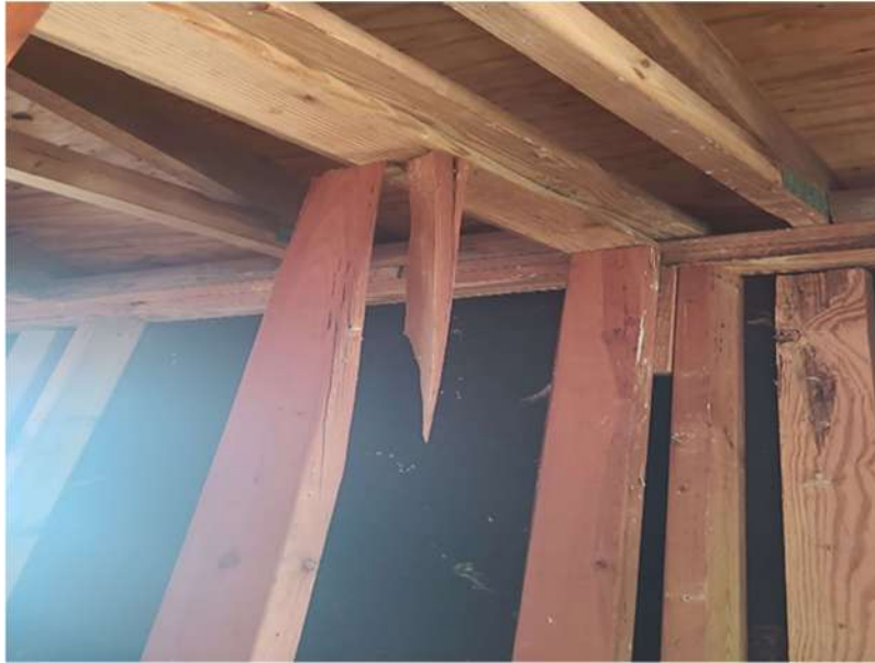
Photo 7: Wall stud broken off from top plate. Broken Member to be replaced.
